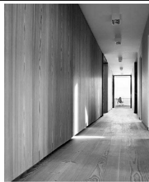
INTERIOR TRIM @ WOOD WALLS NO BASE TRIM AT INTERIOR WOOD WALLS FRY REGLET REVEAL AT BASE
