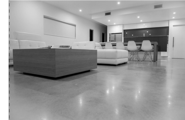
CONCRETE FLOORING - LEVEL 1 FINISHED CONCRETE W/ CLEAR COAT, NO TINT
